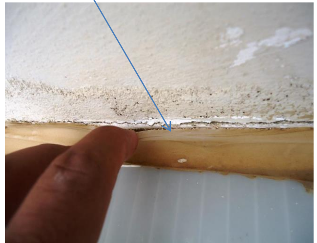
Silicon / not properly fixed
